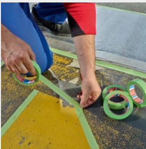
Masking for the coating of floor markings
