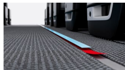
Mounting emergency escape path lighting and floorings: tesa® 45020 removable
