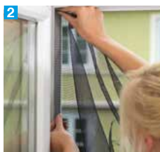
2 Press mosquito net onto the tape
