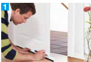
1 Mark the width of the door on the brush
