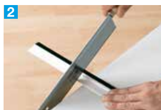
2 Cut the door brush to size
