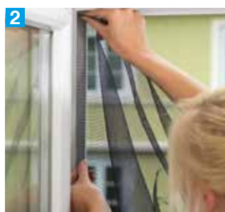
2 Press mosquito net onto the tape
