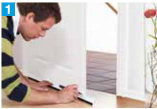
1 Mark the width of the door on the brush
