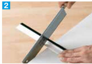
2 Cut the door brush to size
