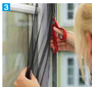
3 Simply cut off excess length
