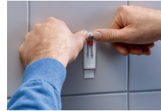
4. Press screw firmly onto the strip.
