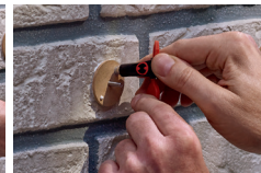
3. Fill in the liquid adhesive and let it dry for 12 hours.
