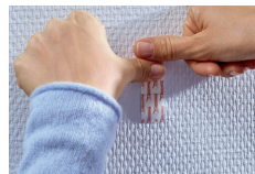
1. Press Adhesive Strip onto the cleaned surface.
