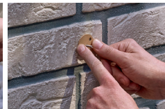
2. Press the screw onto the cleaned surface.
