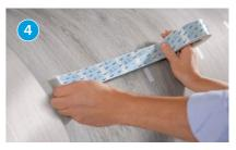
Apply the tape in a straight line, leave a gap of about one thumb's width to the edge of the roll.
