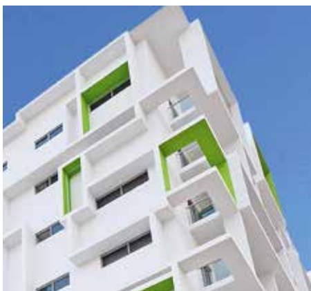
Kube Building Darwin, Australia tesa® ACX plus 70200
