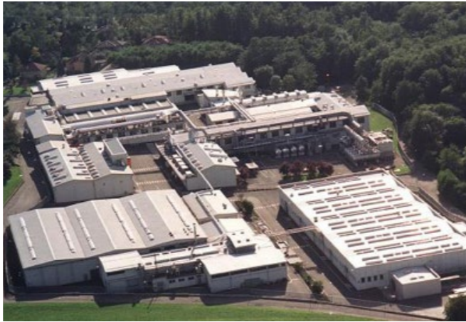
tesa Plant in Concagno
