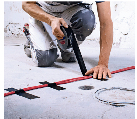
Fixing of cable on rough surfaces
