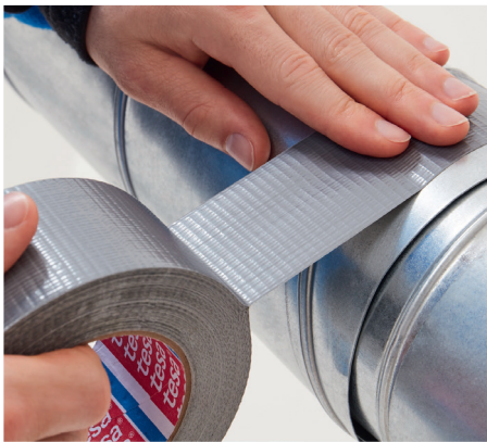
Sealing of ducts
