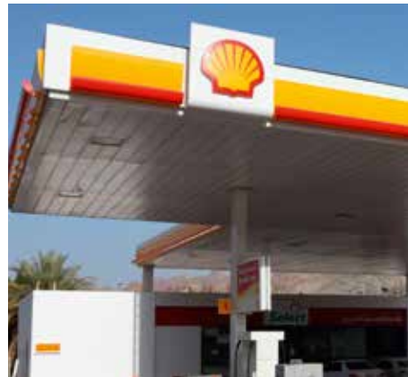
Shell Monolights Kuala Lumpur, Malaysia tesa® ACX plus 7074
