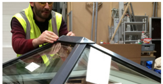
Coping section is bonded
