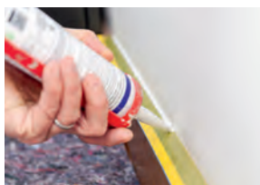
1. Attach, apply filler or sealant
