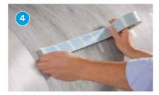
Apply the tape in a straight line, leave a gap of about one thumb's width to the edge of the roll.
