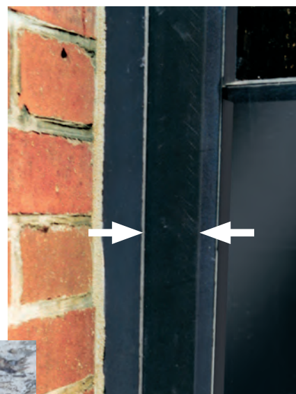
Dark tape mark on weathered anodised aluminium, no adhesive residues
