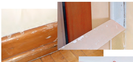
Damage to older varnishes/paint due to excessive adhesion
