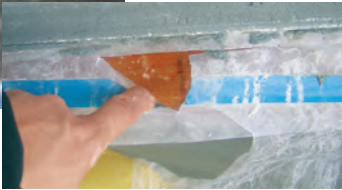
Damaged wood after plaster application. Reason: Masking with insufficiently strong film
