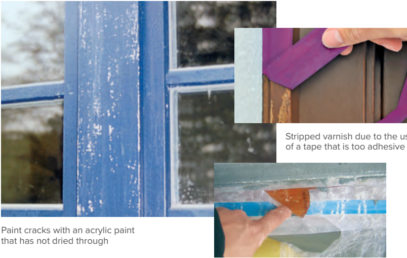
Damaged wood after plaster application. Reason: Masking with insufficiently strong film
