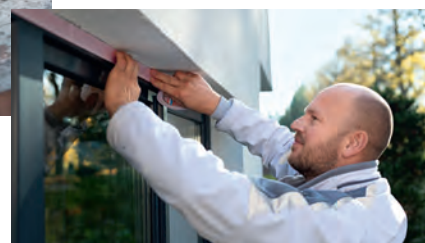
The double-sided adhesive tesa® 4836 makes it easy to apply individual masking
