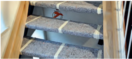
Open stairs: Only use adhesive tape to "strap" around the cover
