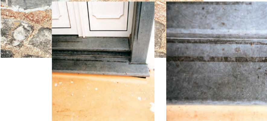
Colour changes to natural stone (Belgian granite, matt finish) after using adhesive tape
