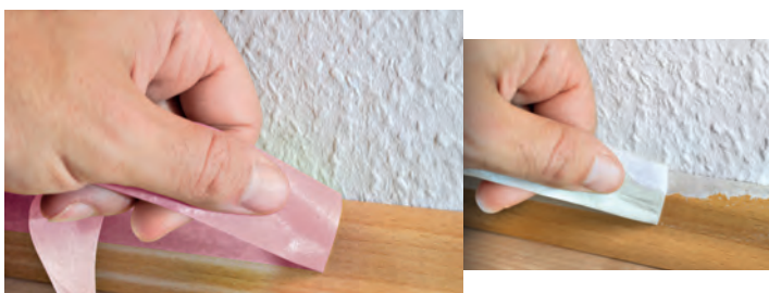
Stripping of the imitation wood; high risk with standard masking tape if removed when wet. No damage with tesa Precision Mask® 4333 Sensitive
