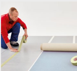
Temporary carpet laying during exhibitions
