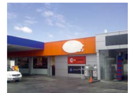
Mogas Heuley Petrol Station Adelaide, Australia tesa® ACX plus 70200
