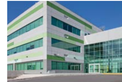
Schneider Building Montreal, Mexico tesa® ACX plus 70200
