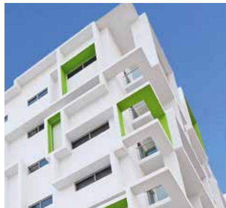
Kube Building Darwin, Australia tesa® ACX plus 7078
