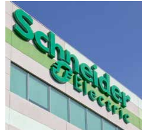
Schneider Building Montreal, Mexico tesa® ACX plus 70200
